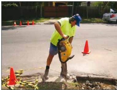
Operating petrol-powered jack hammer
