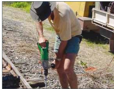
Operating power drill
