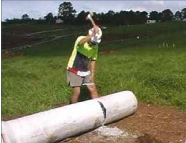
Cutting concrete pipe with hammer
