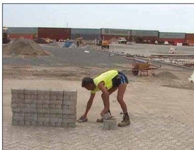
Laying paving blocks
